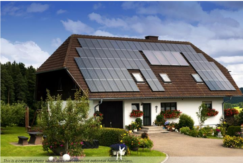
This is a concept photo which does not represent potential home designs.
